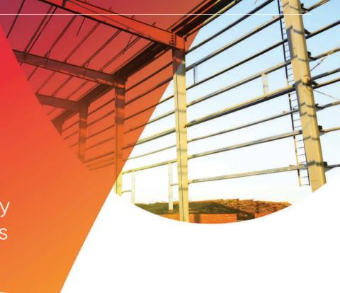
The Heavy Sections sold by ArcelorMittal are produced in accordance with Brazilian Standards "NBR 15980:2024 – Rolled steel sections for structural use – Dimensions and tolerances" and "NBR 7007:2022" – Carbon steels and micro-alloy steels for hot-rolled bars and sections for structural use – Requirements", as well as complying with the main international standards, including the traditional ASTM A572.
